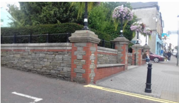
Image 8: Walls, railings & steps to Main Street
